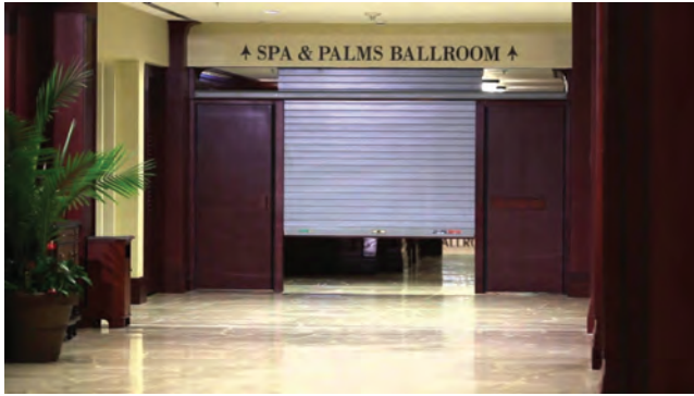
Integrated (T) Type Rolling Shutter Fire Door with Pedestrian Crossing Fire Doors
