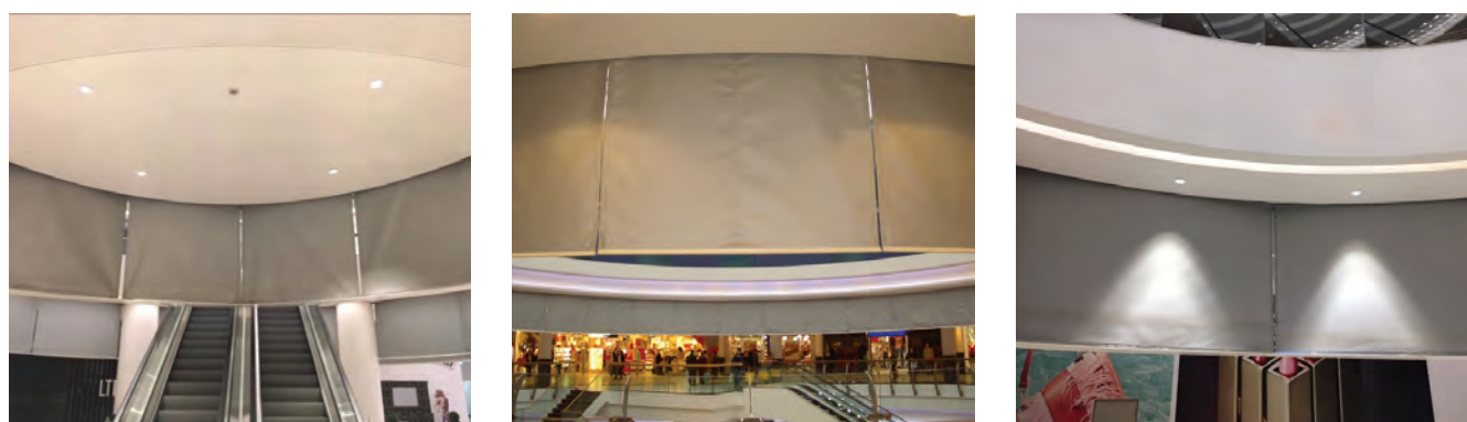
Oval Type Smoke Curtain Applications
