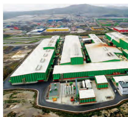
Steel Factory (Turkey)
