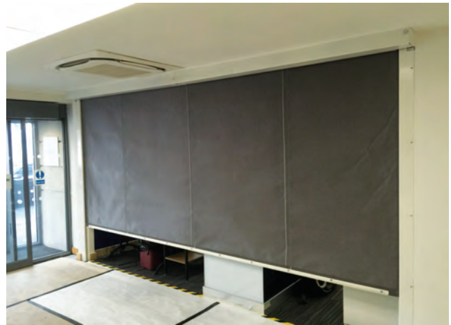
Automatic Vertical Fire Curtain
