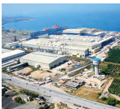
Steel Factory (Turkey)
