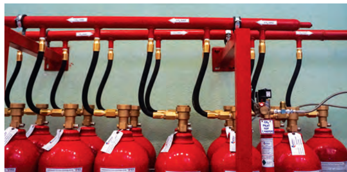
Sample of 200 Bar Inert System
